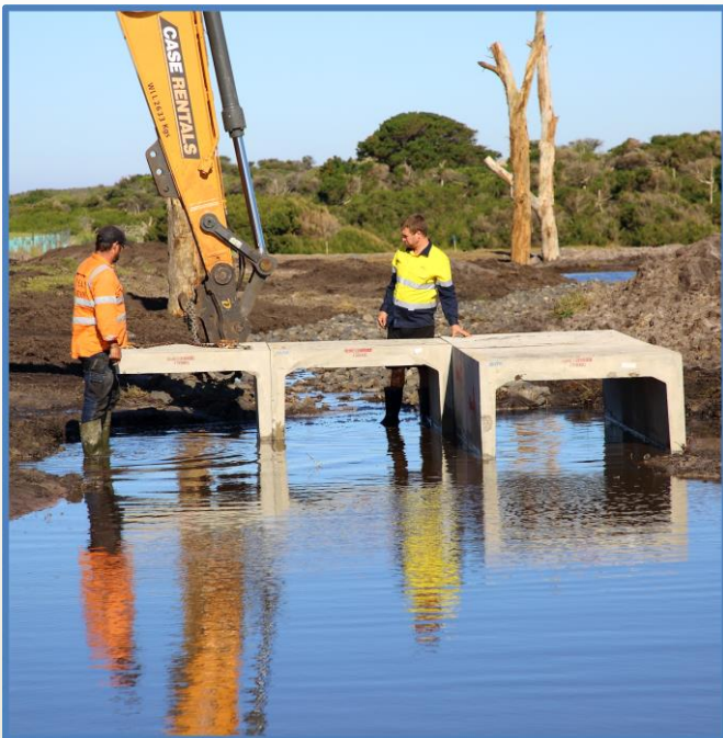
Above: The landscaping lads 'reflecting' on the installation of the culverts in the creek line.
